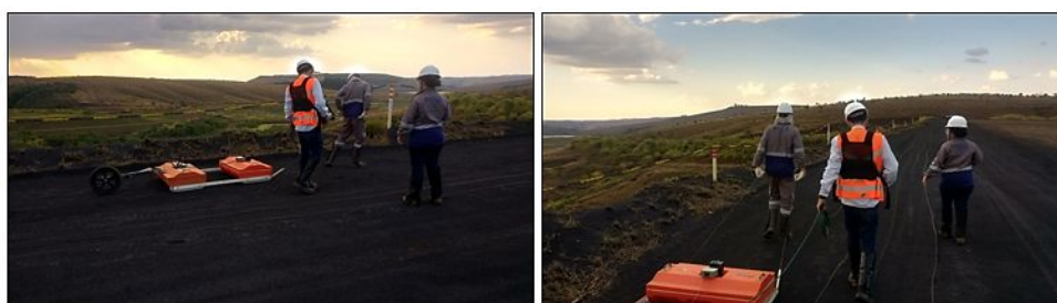
Figure 9 – Acquisition of GPR data at the crest of the BR dam, line L03.
